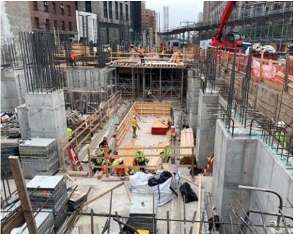
OBP Foundation Construction
