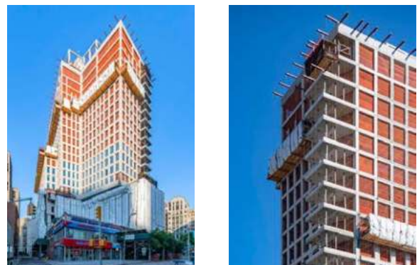
Main Structure & Cantilevered Balcony
