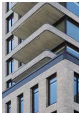
Exterior Brick Details
