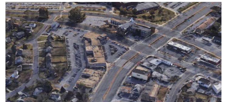
FOUR CORNERS INTERSECTION 2018
