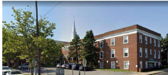
CHURCH EXISTING VIEW
